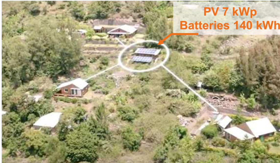
Aerial view of the remote microgrid located in the Circus of Mafate in La Reunion
