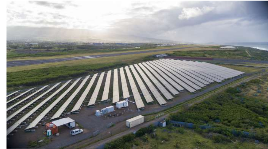
Pierrefonds airport, TotalEnergies (2023) 7.7 MWp PV and 10 MWh energy storage (Picture: TotalEnergies)
